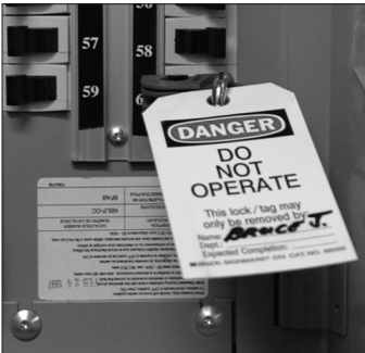
A personal lock with an ID tag—used to prevent other workers from inadvertently switching on an electrical breaker.
