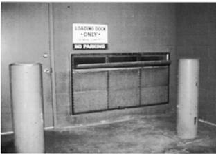
Figure 13: Fresh air intakes inappropriately positioned in a loading dock, can draw toxic fumes into the building's HVAC system.
