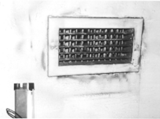
Figure 31: Dirt build-up on supply diffuser.
