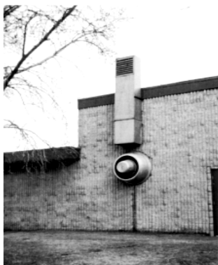
Figure 28: Extension of air intake to minimize cross contamination by building exhaust.
