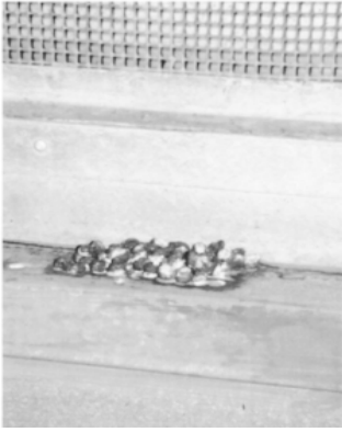
Figure 12: Bird or animal fecal matter near an air intake poses a risk of unpleasant odours and biological contaminants entering the building.
