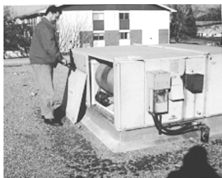
Figure 27: Observe the condition of roof-top mechanical units.
