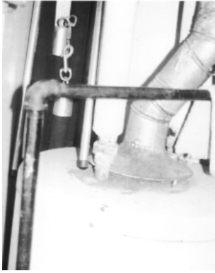
Figure 15: Evidence of backdrafting on a domestic hot water tank.
