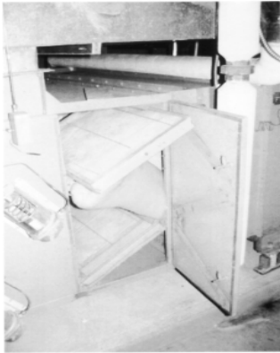
Figure 20: Maintaining and replacing air filters on a regular basis, is crucial for healthy indoor air.
