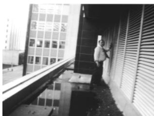
Figure 29: Stagnant water near building air intake.
