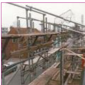
Figure 16. A hoist-console scaffolding
