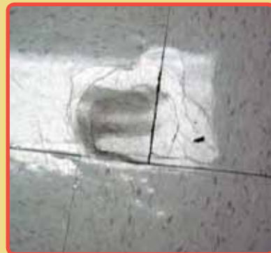
Figure 3.2. Dented vinyl tiles
