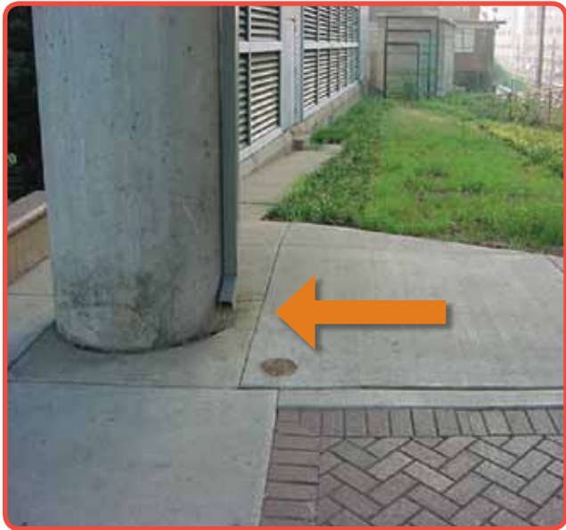
Figure 2.4. Drainpipe routing water onto walkway
