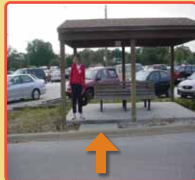
Figure 7.2. Uneven steps by shuttle bus stop, lacking a handrail
