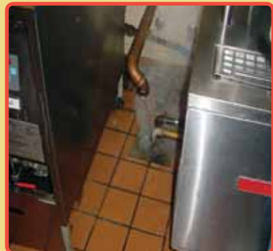
Figure 2.3. Pipe splashing water onto the floor around a drain
