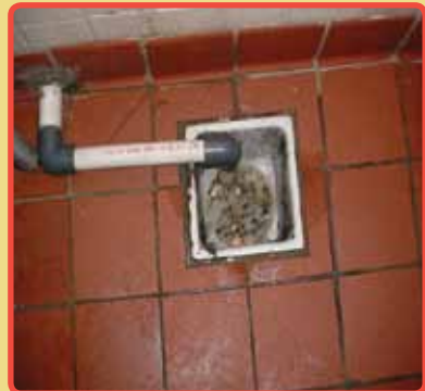
Figure 2.2. Drain is partially clogged with debris
