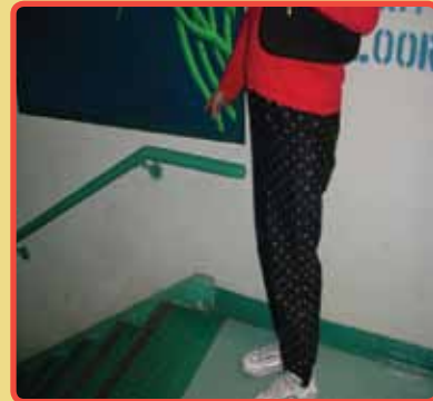
Figure 7.1. Handrail was lowered in order to hang large picture above; handrail too low to be of use
