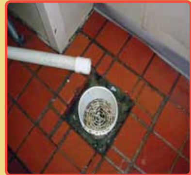
Figure 2.1. Pipe is not aligned properly with the drain causing standing water on the floor
