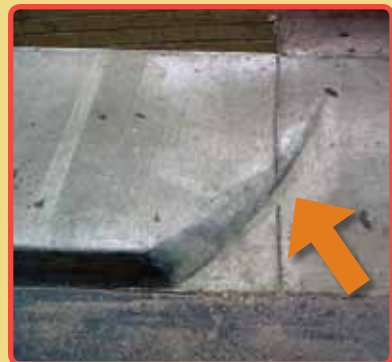
Figure 4.2. Area of sloped pavement that should be highlighted with Safety Yellow paint
