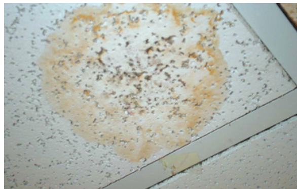
Water damaged ceiling tile with fungal growth
