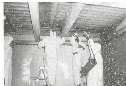
Typical high risk abatement project
