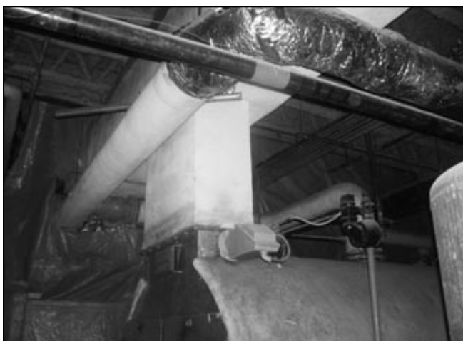
Pipe and boiler insulation
