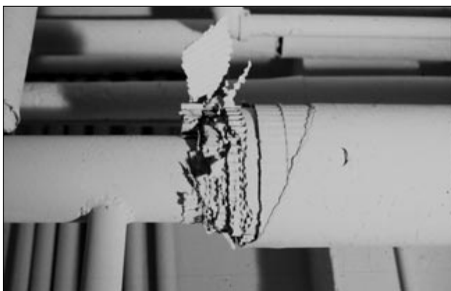
Air cell insulation
