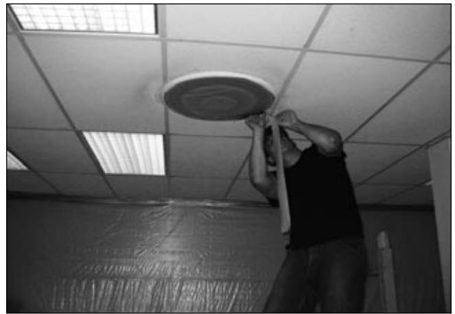
Sealing the ventilation system
