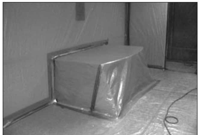
Covered and sealed furniture
