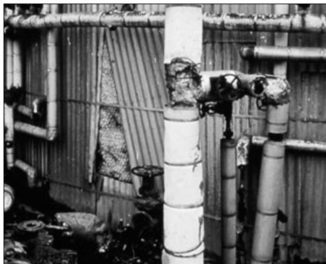
Loose fill insulation
